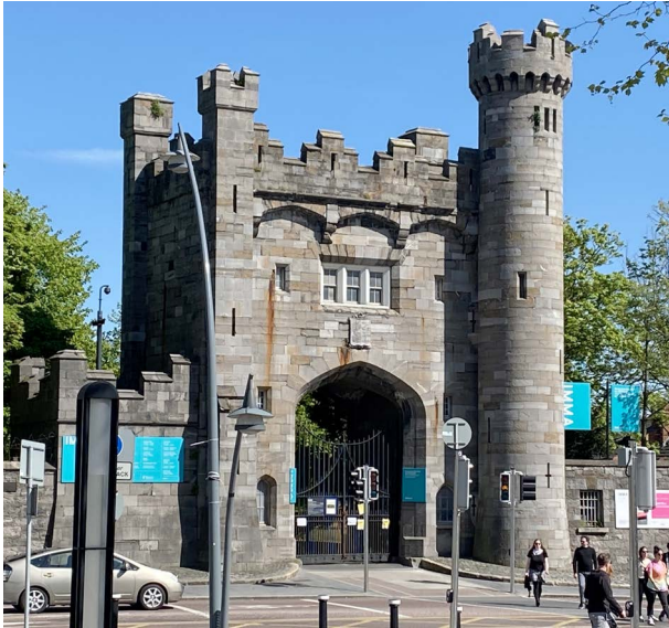
Francis Johnston's Gatehouse
